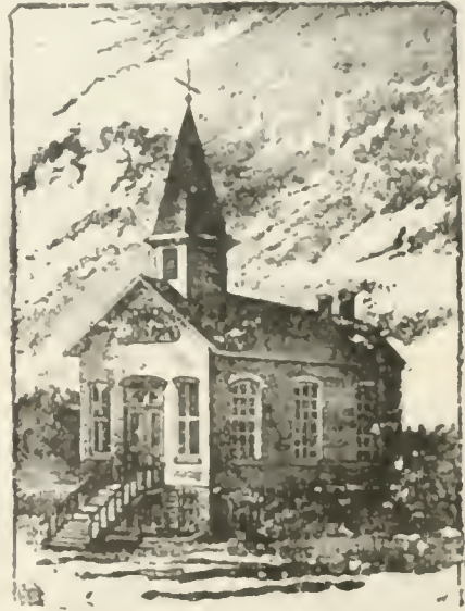
FIRST CONGREGATIONAL CHURCH BUILDING IN OMAHA
